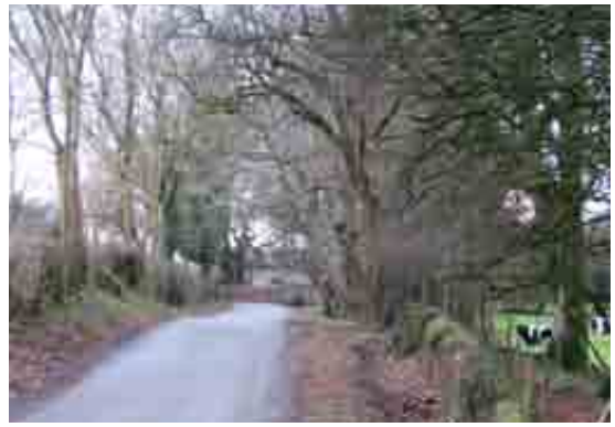
Enclosed and well managed road corridor.
