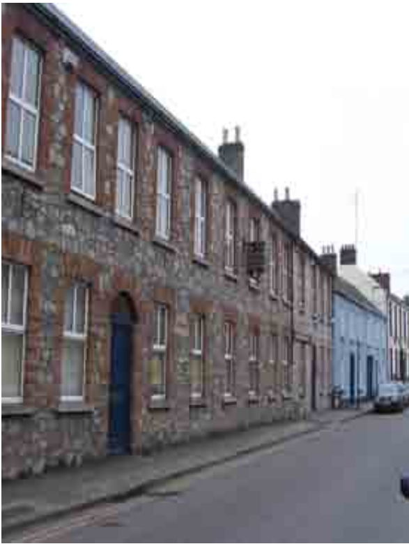
Restoration of historic buildings, Trim
