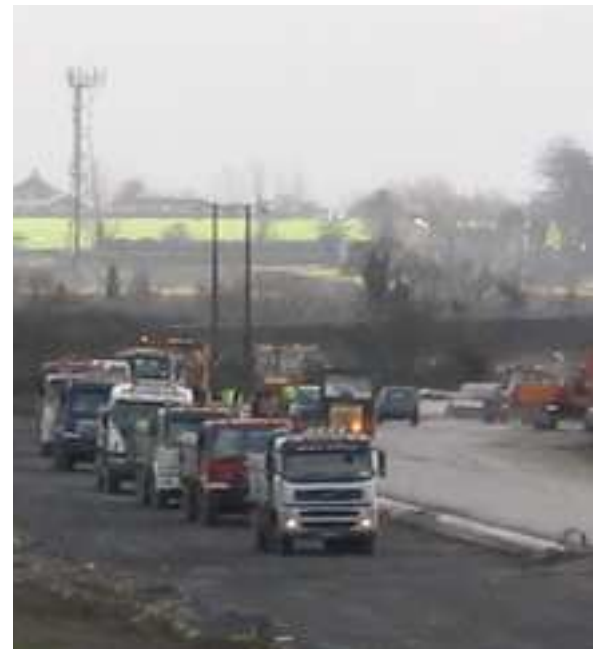
M4 corridor under construction.
