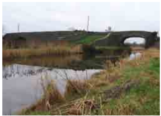
Canal bridge over Royal Canal outside Enfield.
