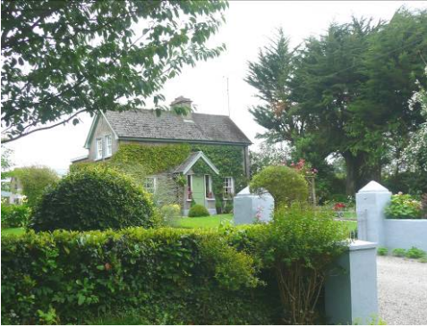
STOREY AND HALF COTTAGE
