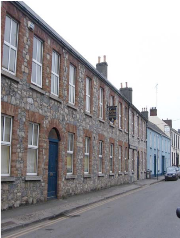
Restoration of historic buildings, Trim
