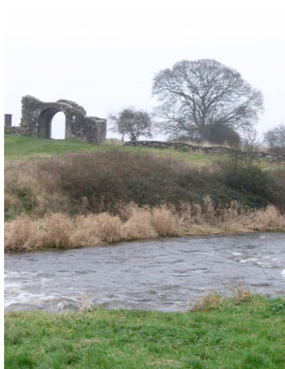
Trim town walls
